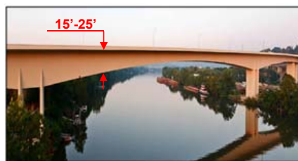
Concrete Segmental Box Girder
