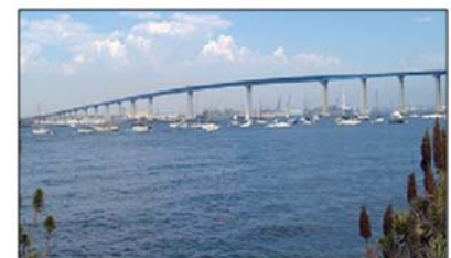
Steel Box Girder
